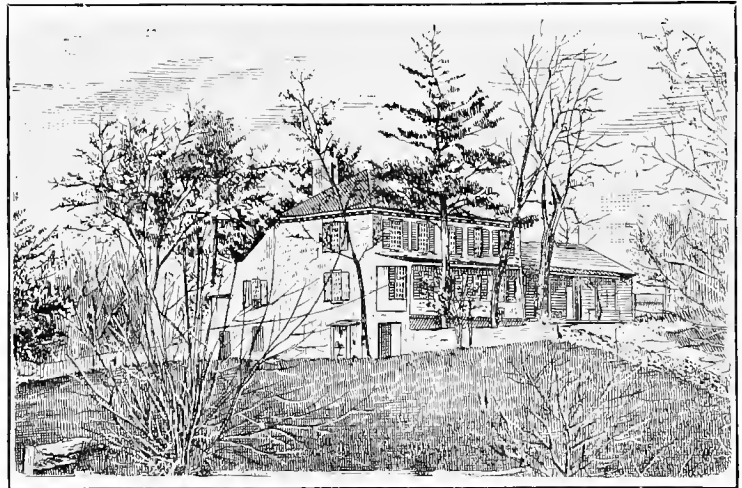
THE JOHN ELLISON HOUSE—Front View from the Old Road.
